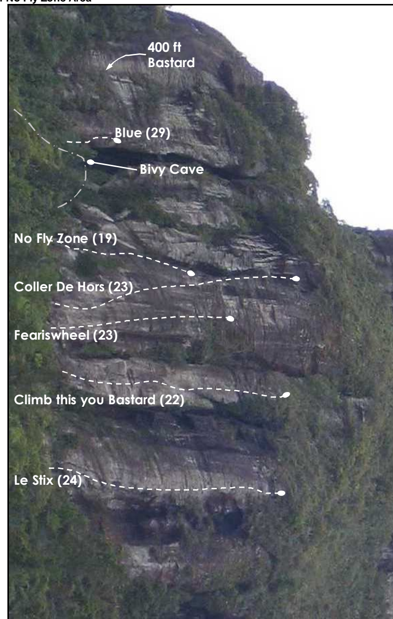
Photo 2: No Fly Zone Area
